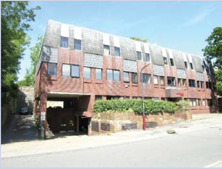
Heathervale House, Vale Avenue, Tunbridge Wells
