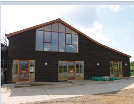
Orchard Business Park, Furnace Lane, Horsmonden
